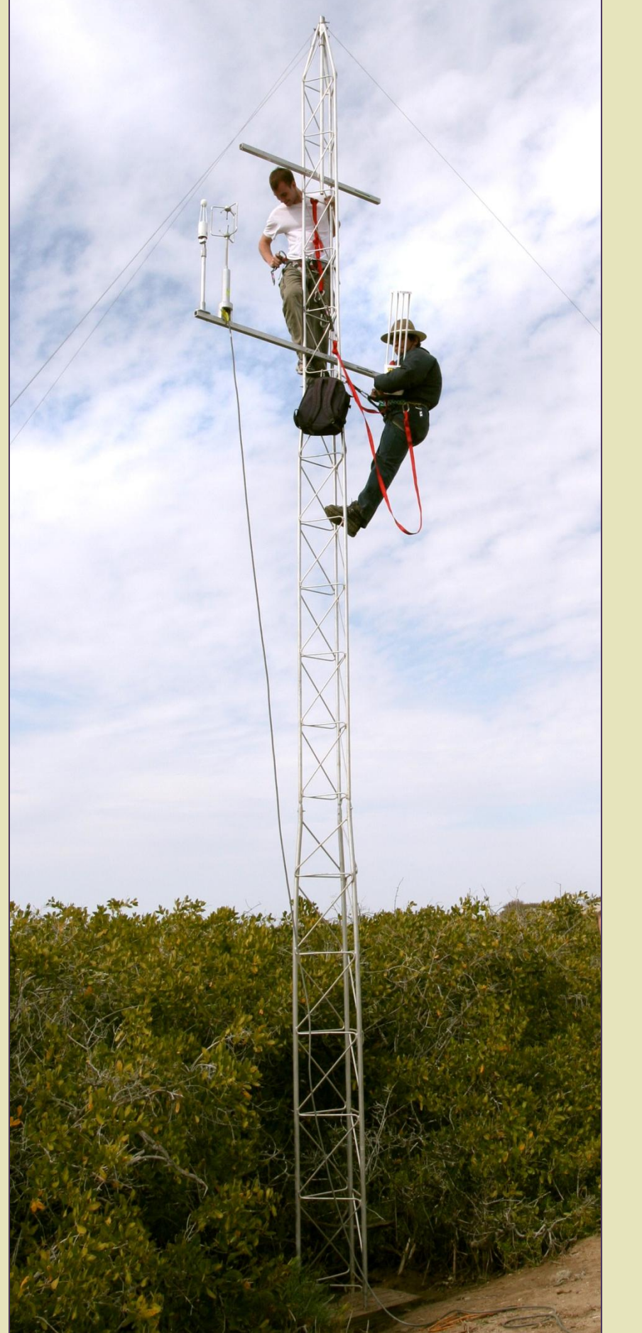
Setting up Eddy Covariance station with LI-7700 and LI-7500 in pacific mangroves, powered by portable generator
